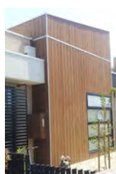
The board shows signs of lightening.
