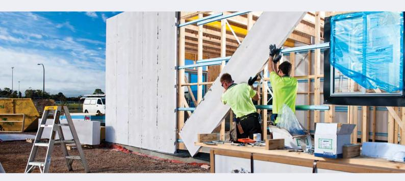
MaxiWall panel is an autoclaved aerated concrete (AAC) steel reinforced, durable, lightweight building panel. The panel has excellent benefits for use in an external wall system for low-rise multi-residential buildings and houses.
