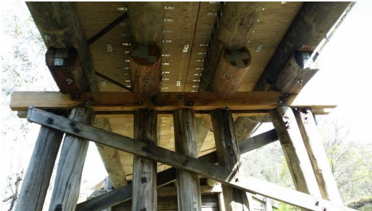
A retrofit solution that can help extend the life of timber bridges by decades, Bridgeply offers a low-cost option for rehabilitating existing, older timber structures without needing to replace the entire bridge – meaning only components that are failing need to be replaced, saving time and material costs.
