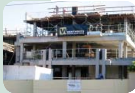
PLYWOOD HOARDING & SCAFFOLDING
