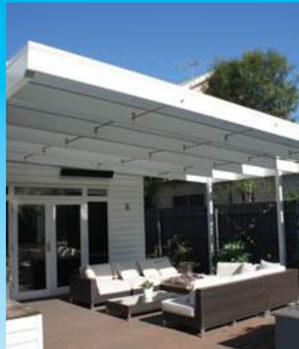
Posts and beams
