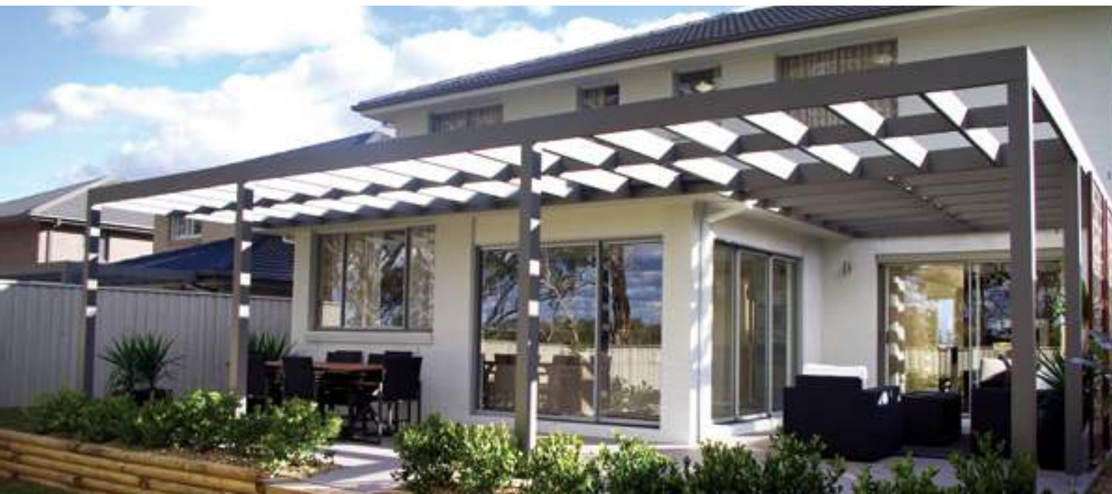
Posts, beams and rafters
