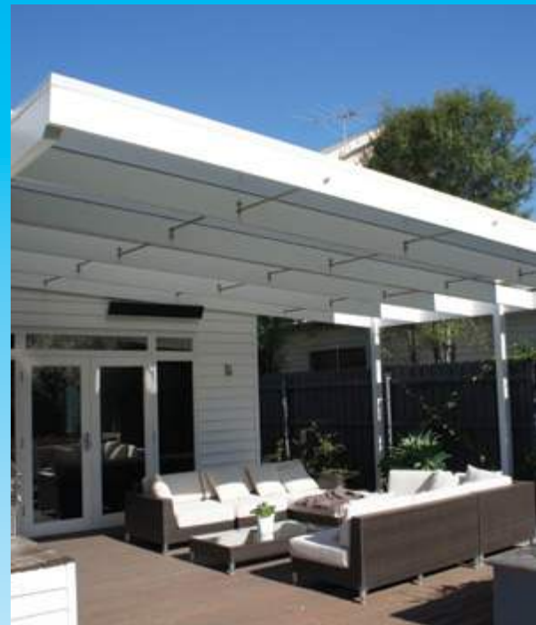
Posts and beams
