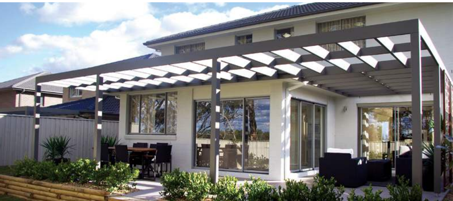
Posts, beams and rafters
