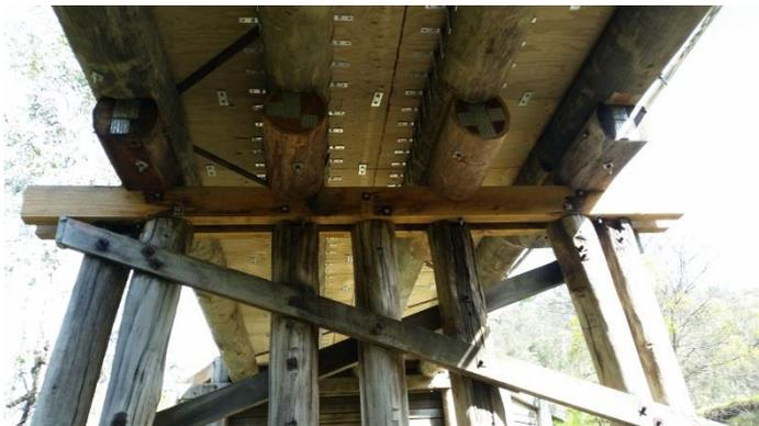
A retrofit solution that can help extend the life of timber bridges by decades, Bridgeply offers a low-cost option for rehabilitating existing, older timber structures without needing to replace the entire bridge – meaning only components that are failing need to be replaced, saving time and material costs.
