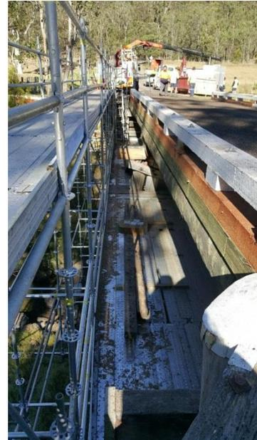
As a way to extend the life of timber bridges, the Cessnock Council selected Bridgeply; a plywood bridge deck system developed by timber specialist and plywood manufacturer, Big River Group. An
